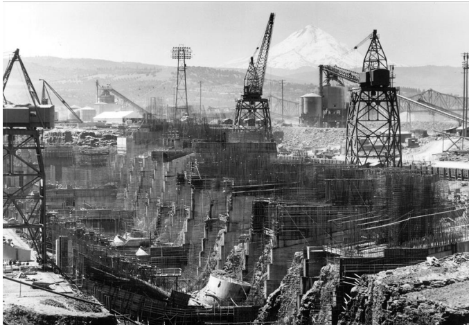
Figure 12: Construction of The Dalles Dam Spillway. Source: Washington State University.
