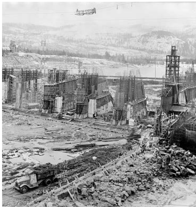
Figure 9: Construction of Bonneville Dam. Source: Washington State University.
